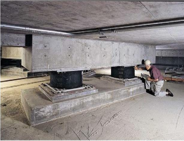
Figure 3: Base isolators
