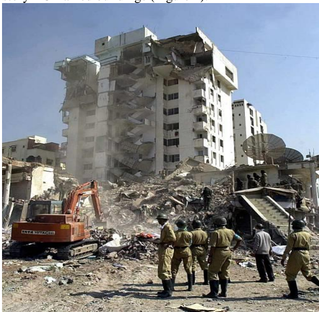
Figure. 2: Apartment collapse in Bhuj (2001) earthquake. ( https://www.gettyimages.in/photos/gujarat-earthquake )
