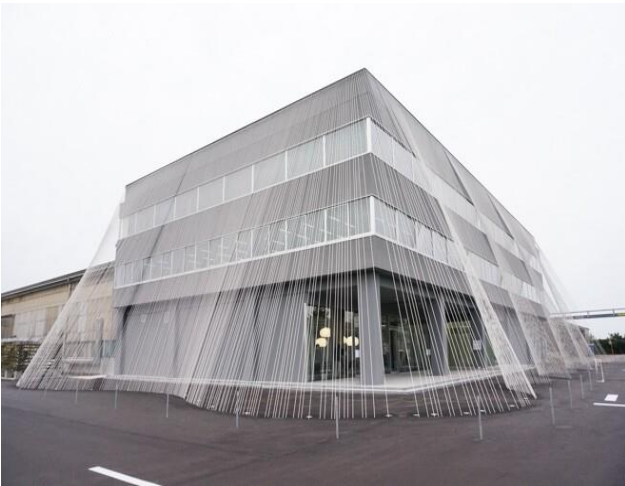
Figure 4: Structure made with carbon fibre material in Japan
