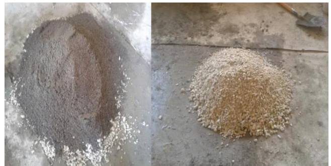
Figure 2: Mixing of concrete
